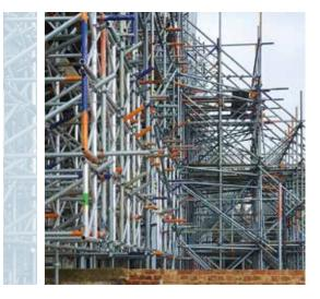
The scaffold temporary works have been continuously monitored and amended throughout the project, due to the complexities of the exposed building and the requirement to meet the ever-changing calculations.
